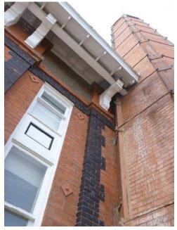
Figure 2: Exterior construction is composed of multi-wythe brick walls with a concrete section on top supporting the roof framing. The smokestack is free-standing above the roof line.
