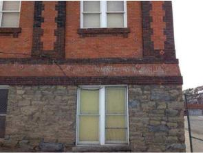
Figure 9: Evidence of settlement at the northeast corner of the building includes cracking in the rubble-stone foundation (left) and the exterior brick (right).
