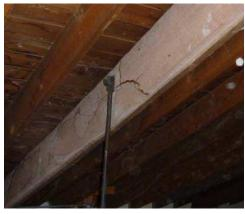
Figure 11: Cracked rafter at hanging track mezzanine connection.
