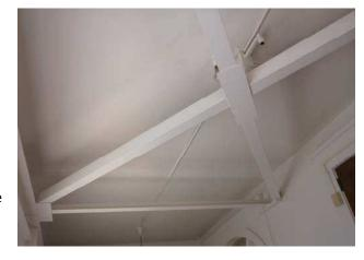
Figure 6: Cross-bracing at entry stair.
