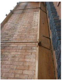
Figure 8: Steel framing retrofits at exterior smokestack.
