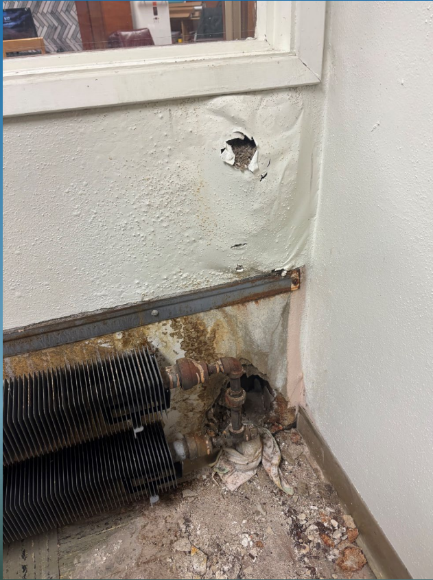
Failed condensate return pipe in library
