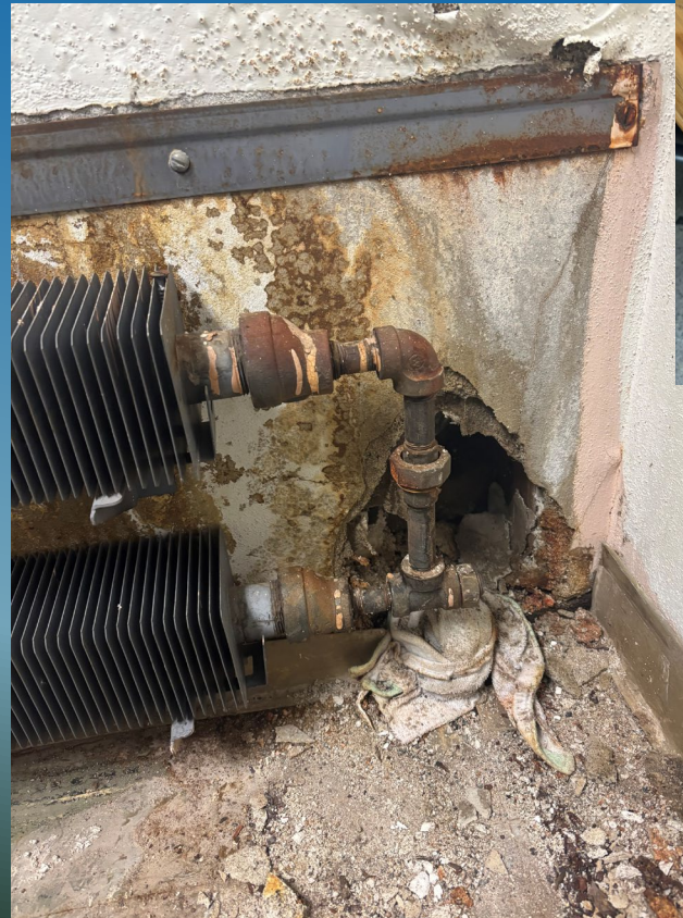
Failed condensate return pipe in library
