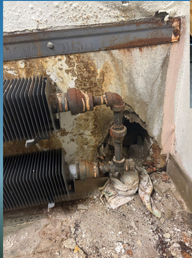
Failed condensate return pipe in library
